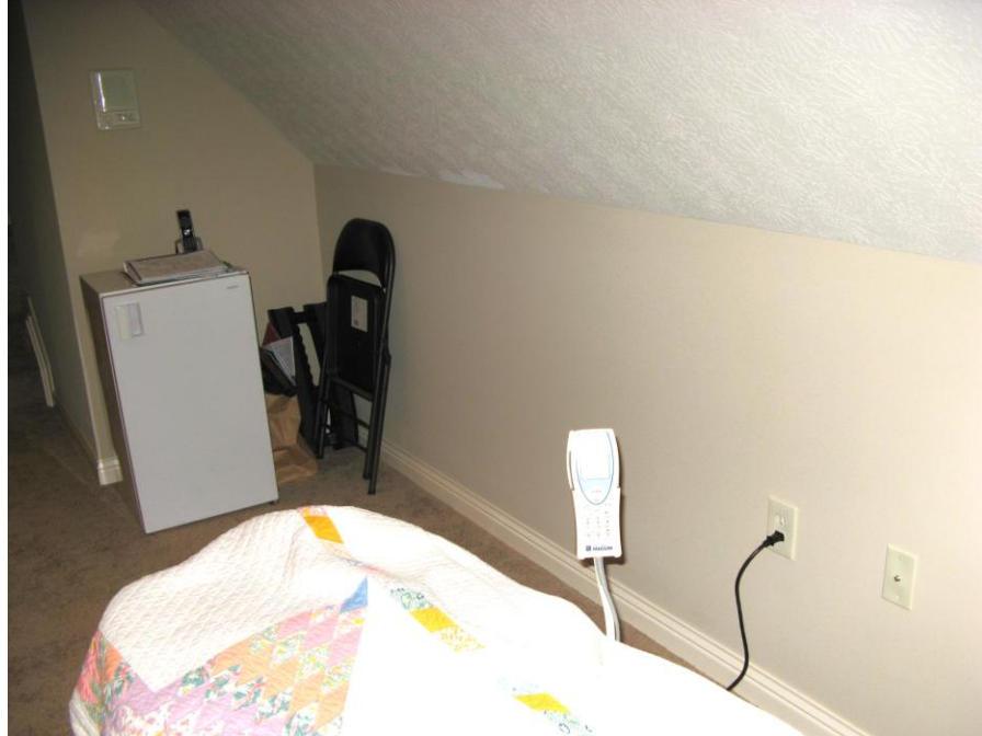
B. Photograph indicates area in which above thermogram was recorded - Bonus Room, east elevation.
